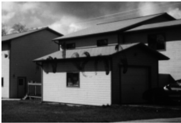
Morton Street Casino
