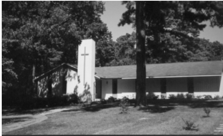
Pineville Presbyterian Church is an Orthodox Presbyterian congregation.
